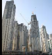
URBAN INFRASTRUCTURE & HOUSING
