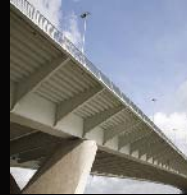
ROAD BUILDING & ROAD RECYCLING
